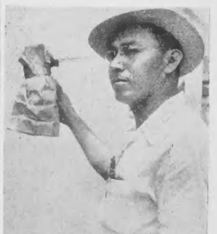
MONEY-SAVER. H. V. Tromp, subforeman in the M & C Paint Department, points to a time-saver - and thus money-saver - idea of his which is now in use. Paper bags held in place with rubber bands are placed over electric light bulbs to protect them while paint is being sprayed in the vicinity. It is estimated that this new method requires only 1/3 of the time required by the old method of coating the bulbs with a layer of grease.
